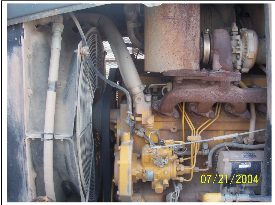
Compressor mount area
